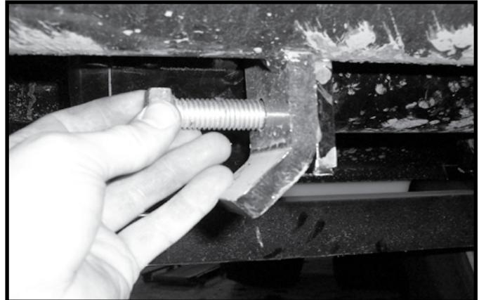
7. Using fork lift, lower tank assy down onto bearing assy. Install 3/4" bolts on bearing assy. Leave bolts loose.
