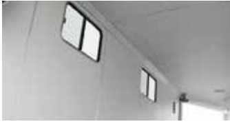
Windows, White Luan Walls and Ceiling
