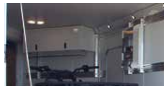
Combo Walls, Gear Cabinets and Racks
