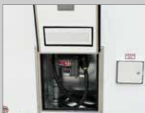
FUEL STATION WITH ACCESS DOOR AND 30-GALLON TANK
