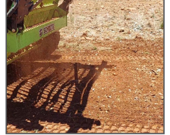
The area behind is left clean, of stones from 2"-27" (5cm - 69cm)
