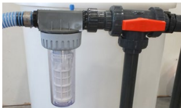
Heavy duty filter and 3-way valve
