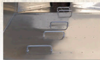
Inside Hopper Round Bar Ladder
