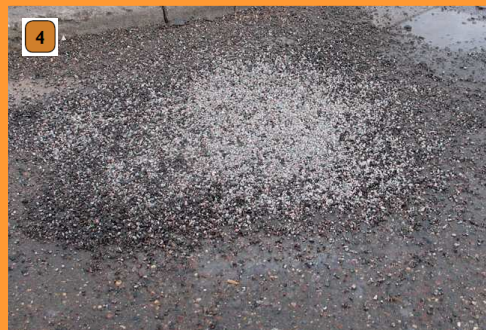
Spray dry aggregate as cover material.
