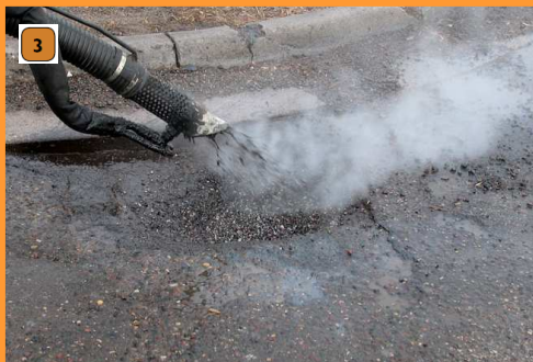
Spray inject the mix emulsion/aggregate.
